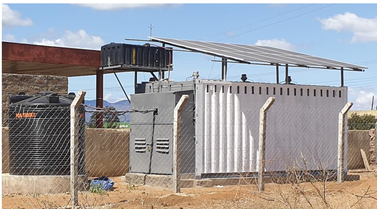
Figure 4. A forced-air evaporative cooling chamber constructed by MIT D-Lab and Solar Freeze, near Kibwezi, Kenya. This chamber has a storage capacity of 168 vegetable crates (> 3,000 kg of produce) and is fully powered by the solar PV panels (above the chamber) and a battery storage system. This chamber is used by farmers and vendors who pay a fee to store their produce in the chamber.
